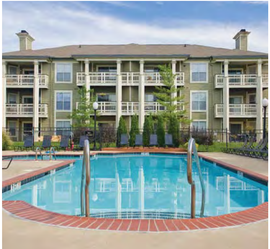
Windsor at Windemere Place in West Chester, PA. Apartment community offering short term and long term lease.
